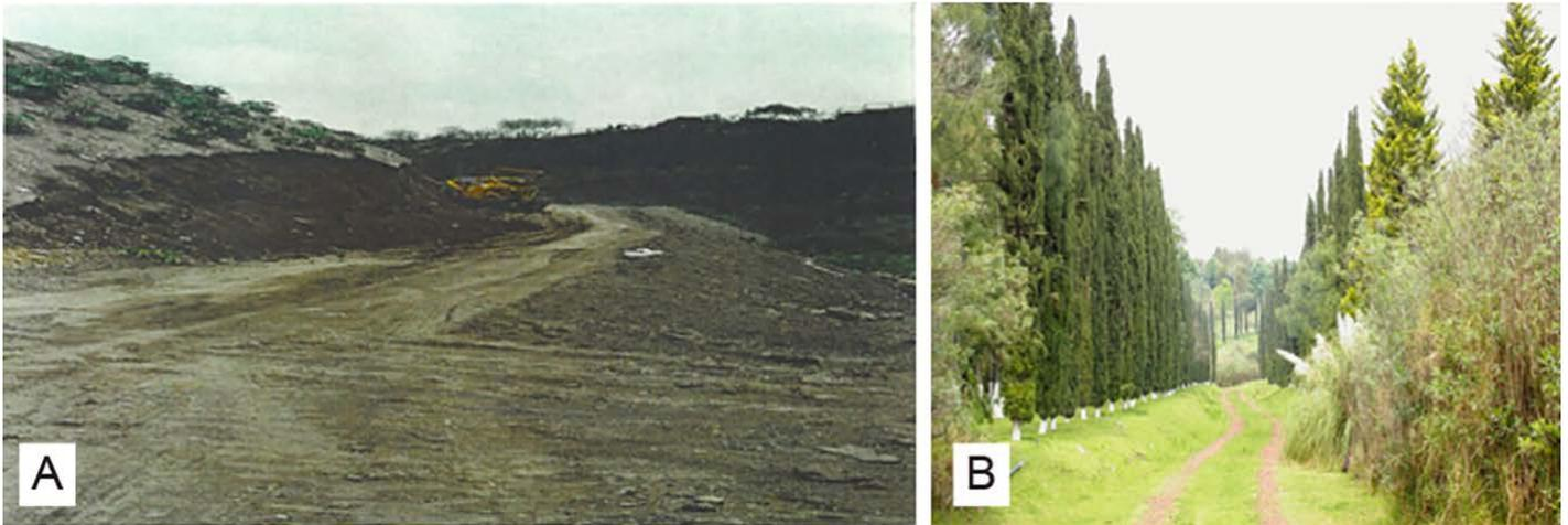
Figure 18. A. Movement of the material deposited in the quarry to stabilize the slope forming terraces for subsequent revegetation and outlining the access road that was built afterwards. Courtesy of Francisco Martínez, 1997. B. Exotic trees which were planted on the terraces. Courtesy of Manuel Figueroa Maheng, 2006.
